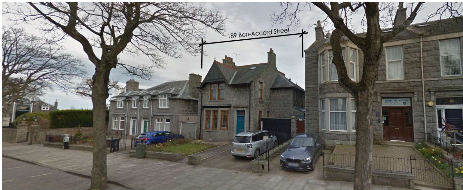
View from Bon-Accord Street showing extent of proposed dormer visible
